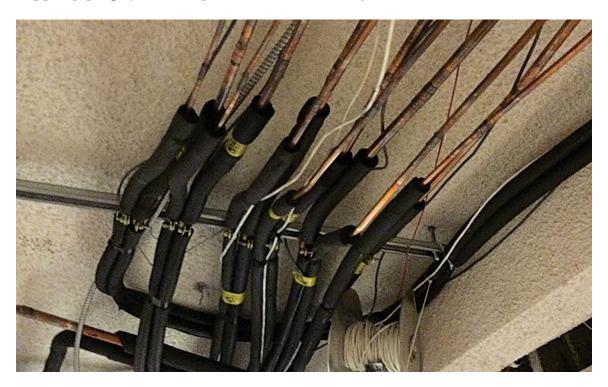
**Figure 3** shows some of this tubing being installed in the hallway of a commercial building. A multistory building with such a system could contain several thousand feet of copper tubing with hundreds of brazed or mechanical joints. Hydronic systems can use larger piping for mains and thus reduce the linear footage of piping and joints that needs to be installed.
